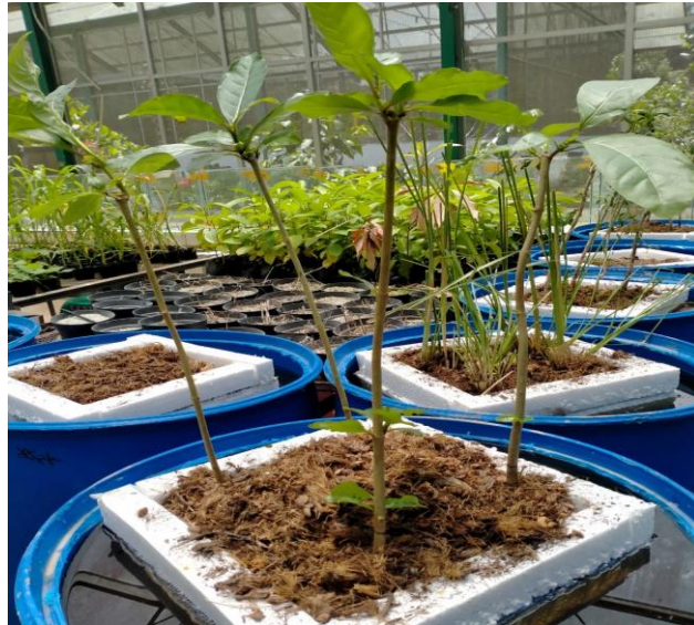
Figure 16 Floating treatment wetland
